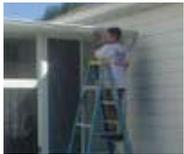
**Step 4: Priming.** Priming bare wood and metal will be done with appropriate primers. Horizontal areas where water may sit creating rusting areas will be given two coats of primer.
